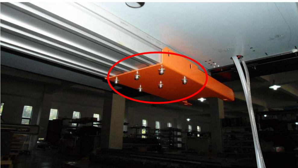
Remove shipping bracket fixing screws, and remove Orange brackets.
